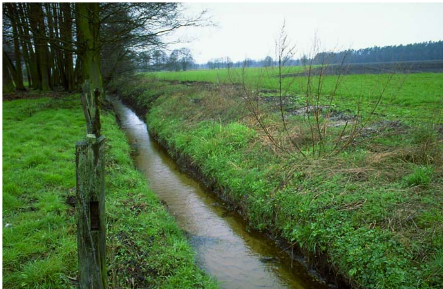
Fig. 4: The Endeholz Ditch in spring of 1998 after management by machines. On the right side the excavated material can be seen. The river bottom is exclusively sand. The ripples are characteristic of the moving sand.
